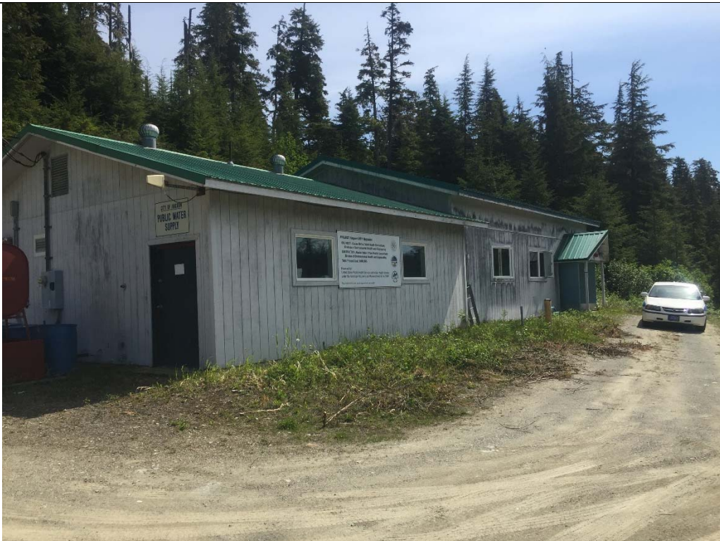
Treatment plant building.
