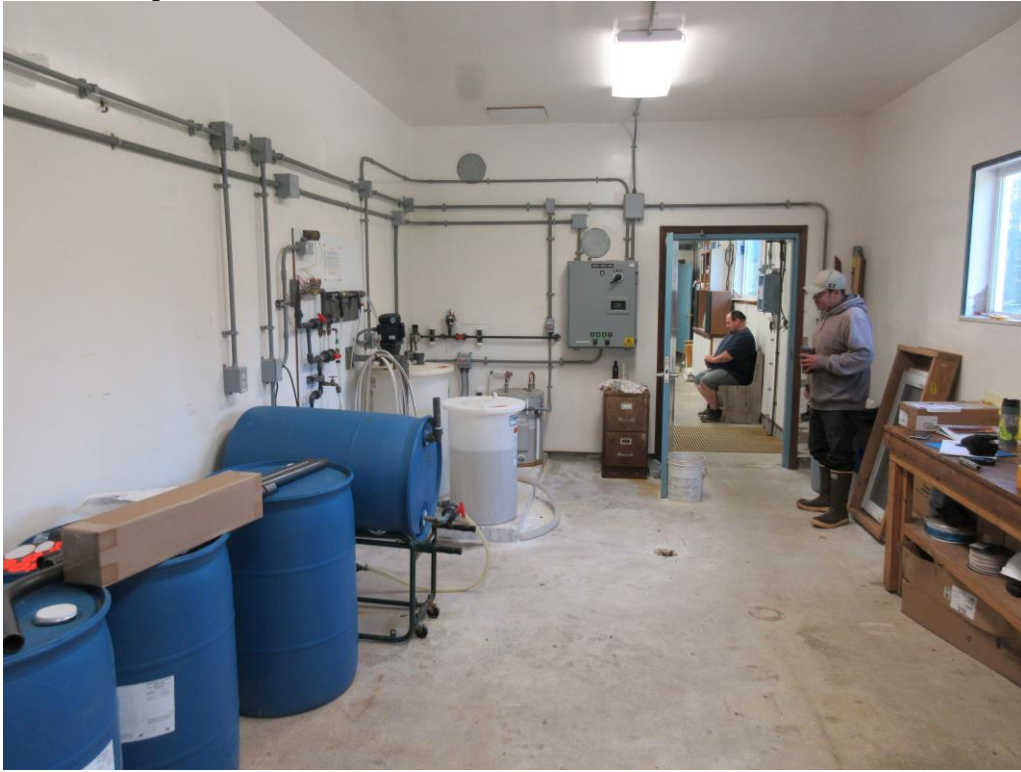
entrance to plant:
