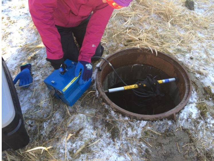
Figure 2: Flow Monitoring Upstream of Settling Tanks
