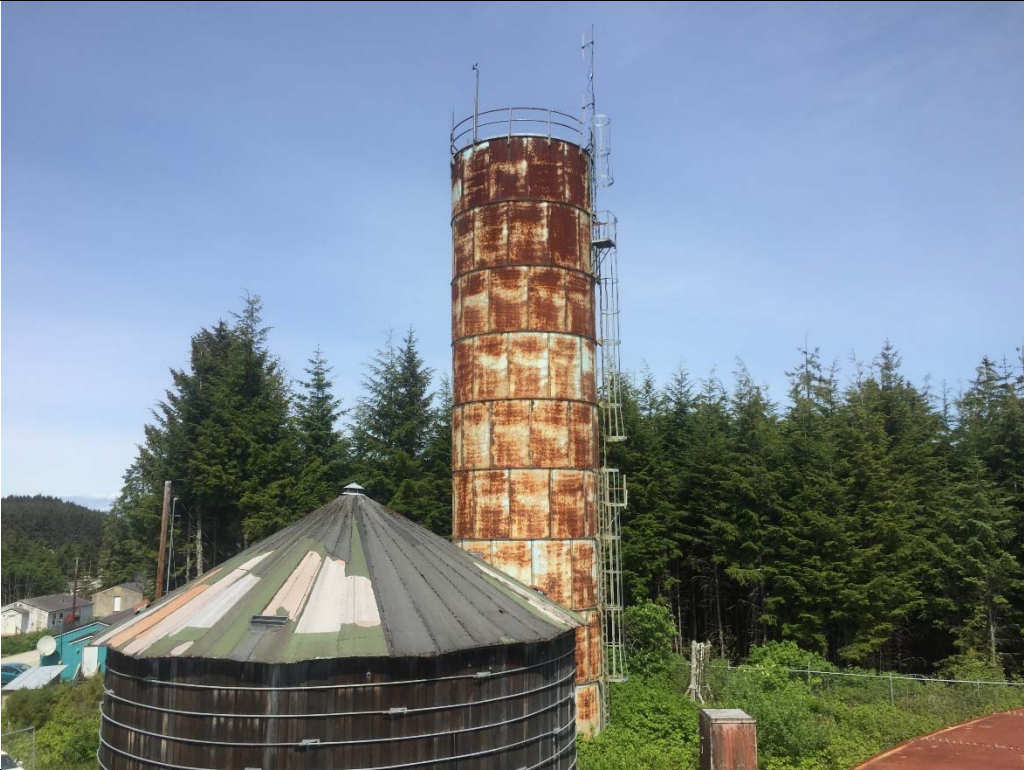
150,000 gallon standpipe, viewed from roof of second 500,000 gallon tank.
