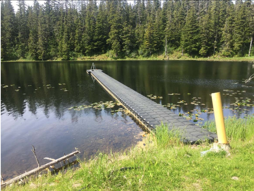
Raw water intake structure.
