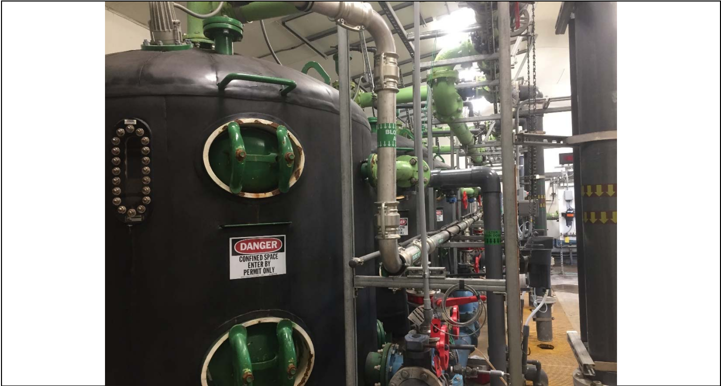
Filter #4 in foreground was out of service during survey for maintenance.
